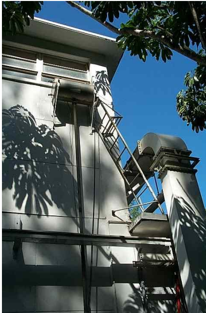
Water storage tank on side of building. Note the waveguide, leaving the EH tuner on the mezzanine and heading down to loop beneath the road.
