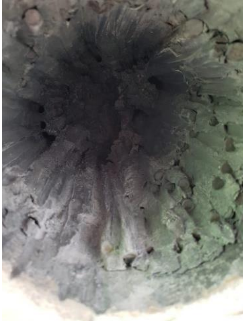
Figure 6.0-2. Wire Strands inside Failed Socket
