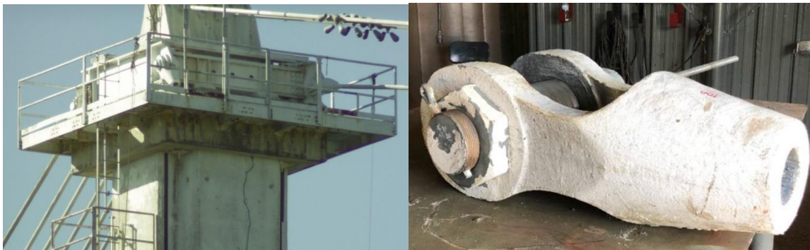
Figure 6.0-1. Tower 4, including Socket
