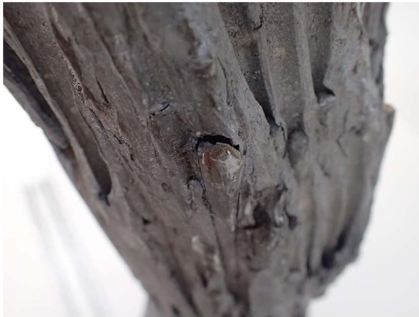
Figure 156. Close up view of a wire fracture on the 2 o'clock side of the cable-end section.
