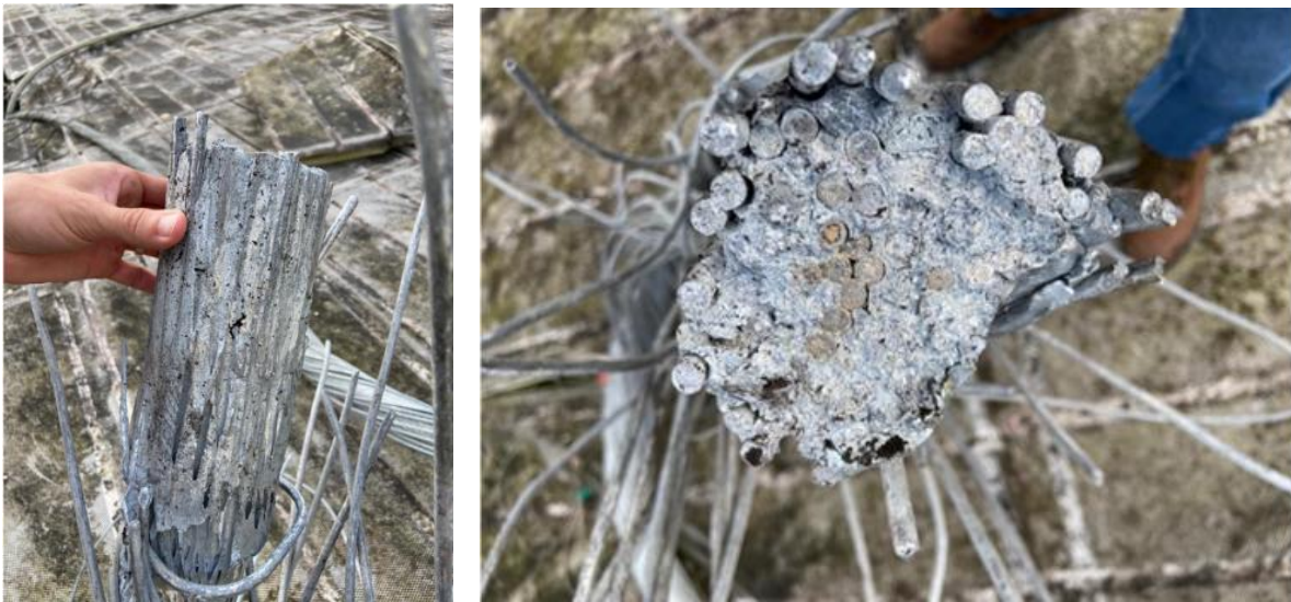
Figure 6.0-3. Pulled-Out Cable Wire, Strands and Zinc (side view)
