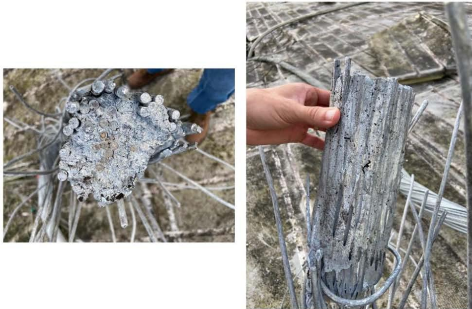
Figure 11. Photos of the failed M4N auxiliary cable-end from the Tower T4 socket connection. These photos were taken prior to the ultimate collapse of the observatory. The cable was not retrieved from the observatory site until after the ultimate collapse of the observatory. Photos provided by WJE.
