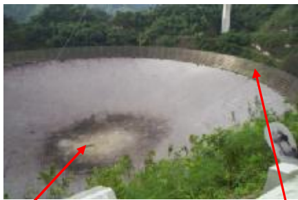
View of the 1,000-foot reflector showing the center hole and the 50-foot-high ground screen along the outer edge of the reflector.
