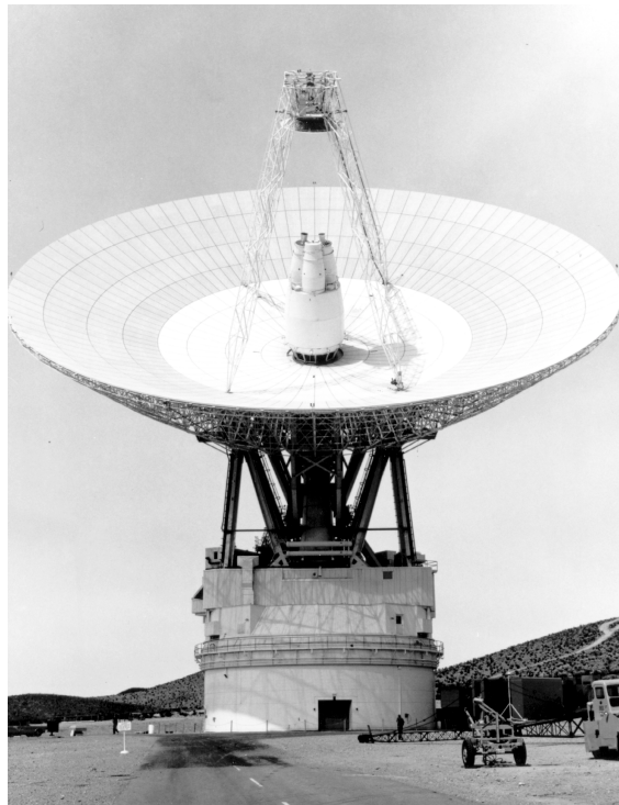
Fig. 5-9. Tricone installed on the 64-m antenna.
