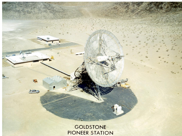
Fig. 2-4. The Cassegrain installation at DSS-11.
