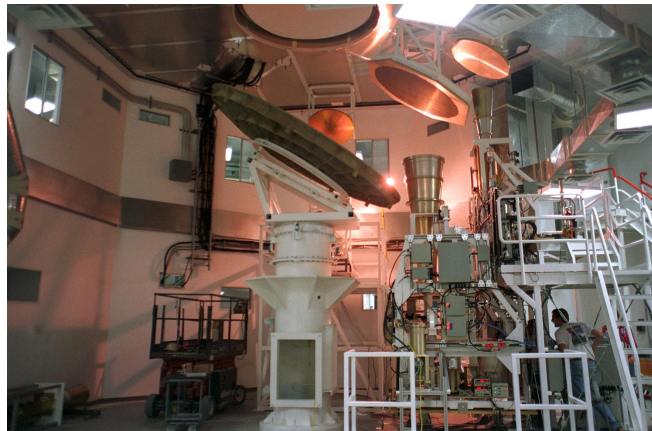
Fig. 8-8. The S-/X-band feed system at DSS-24.
