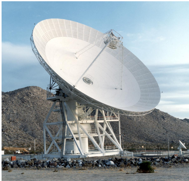
Fig. 7-37. DSS-13 after bypass beam-waveguide removal.
